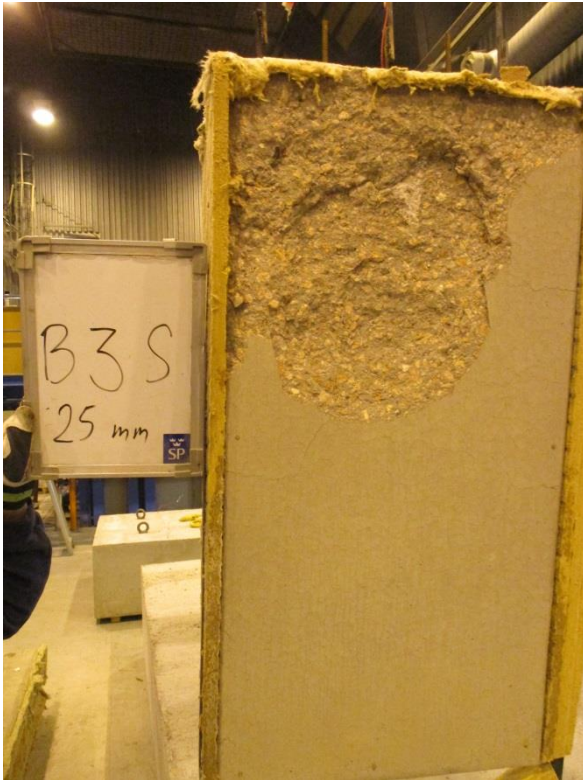
Figure A66. Test specimen Wedge-Slab 21: 1000x500-50-300 Mix 2 0.33-0.0kgPP after the test. Maximum spalling: 25 mm
