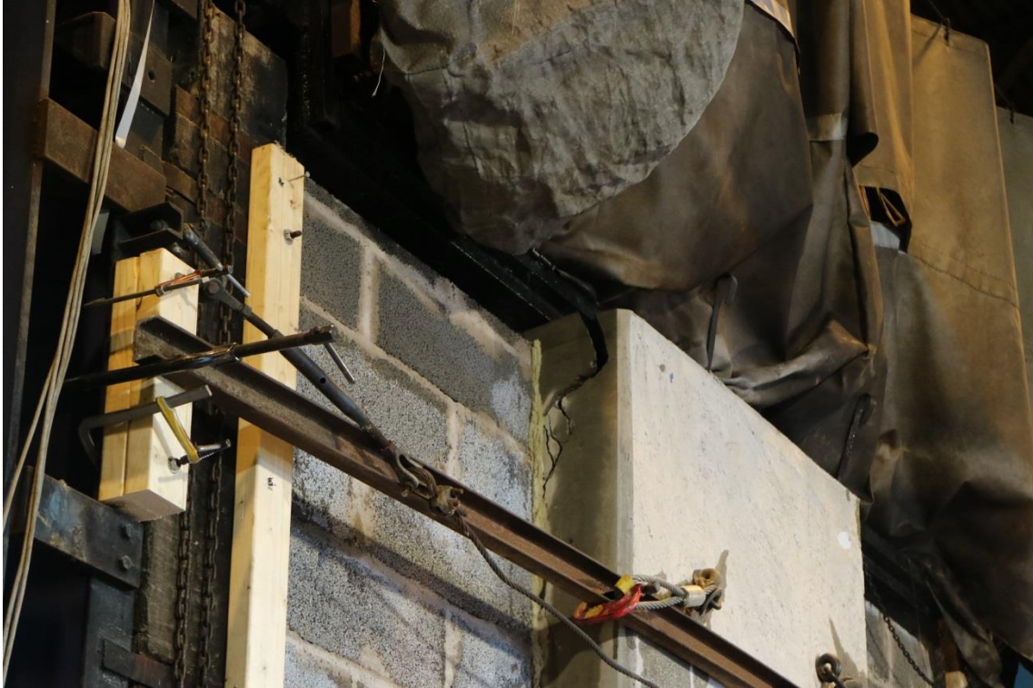
Figure A156. The slab is cracked at the top.
