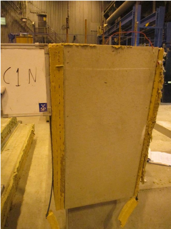
Figure A69. Test specimen Wedge-Slab 22: 1000x500-50-300 Mix 3 0.40-0.0kgPP after the test.
