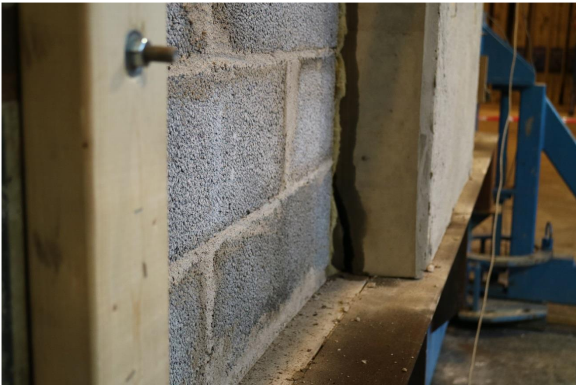
Figure A155. The slab is cracked at the bottom.
