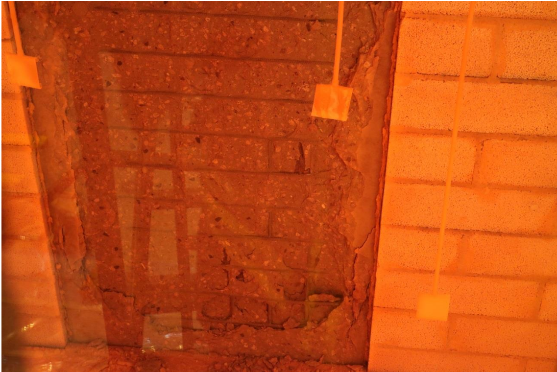
Figure A154. The fire exposed side after 39 minutes of the test.
